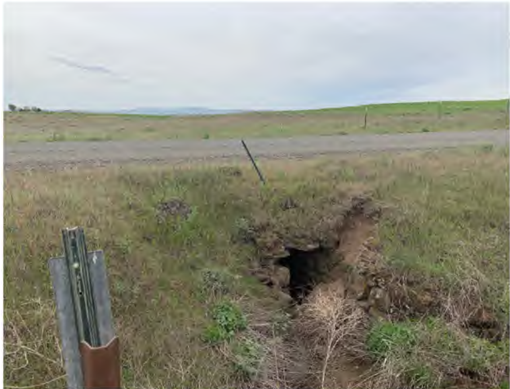
Photo 24: Culvert 4, approximately 36 inches in diameter and made of brick.
