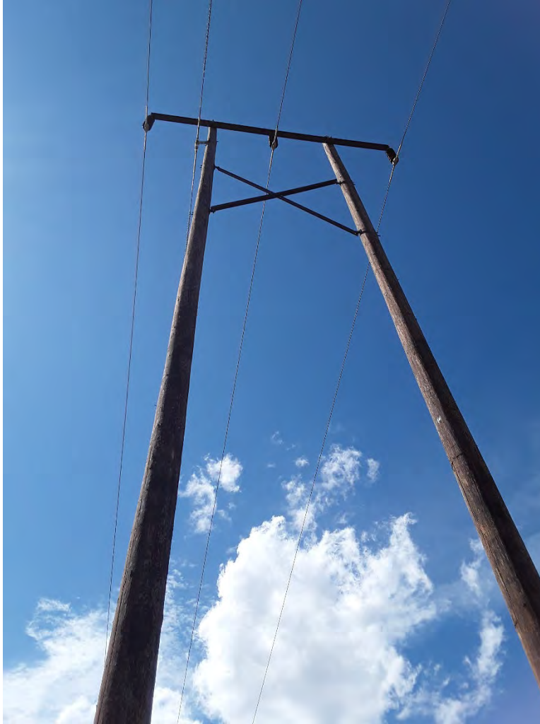
Photograph 13. Midway-Moxee Transmission Line (Site 676383) wood pole structure, conductors, and fiber optic cables.
