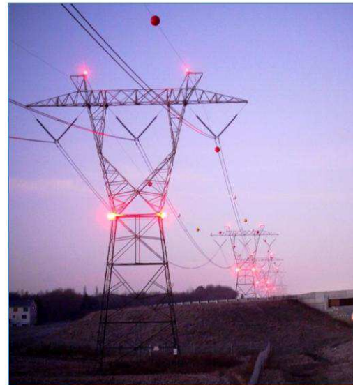
Figure 3: Monitoring-only sites alongside NJ Turnpike, NJ on cellular/radio hybrid network.
