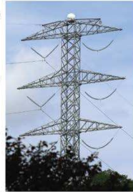
BELOW: HARRIER Utility tower installation
