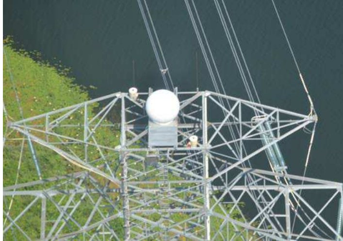
Figure 4. DeTect X-Band ADLS Radar With Radome Enclosure
