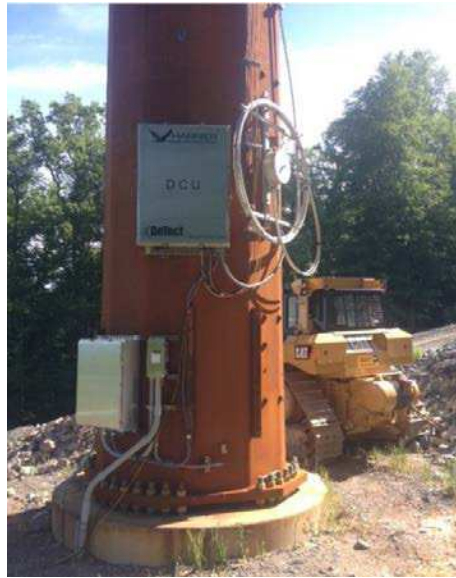
Figure 15. The DCU Installed on Transmission Tower [6]
