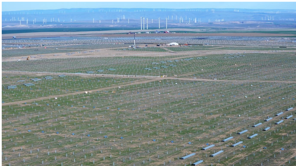
Photo 14. Early phase construction of USSE in Gilliam County, Oregon, May 2022. Racking systems (white posts) are installed with solar arrays staged nearby. Wind energy turbines in the distance.
