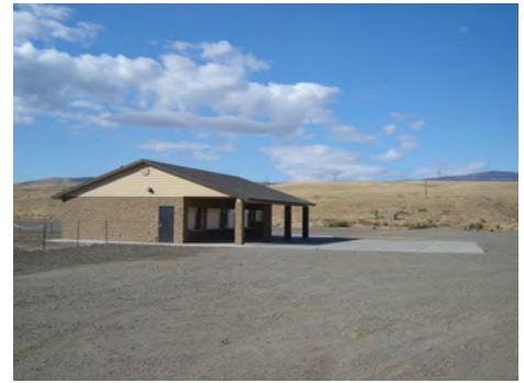
Figure 23 - Landscaping could help blend improvements into the surroundings in Horn Rapids and other parks
