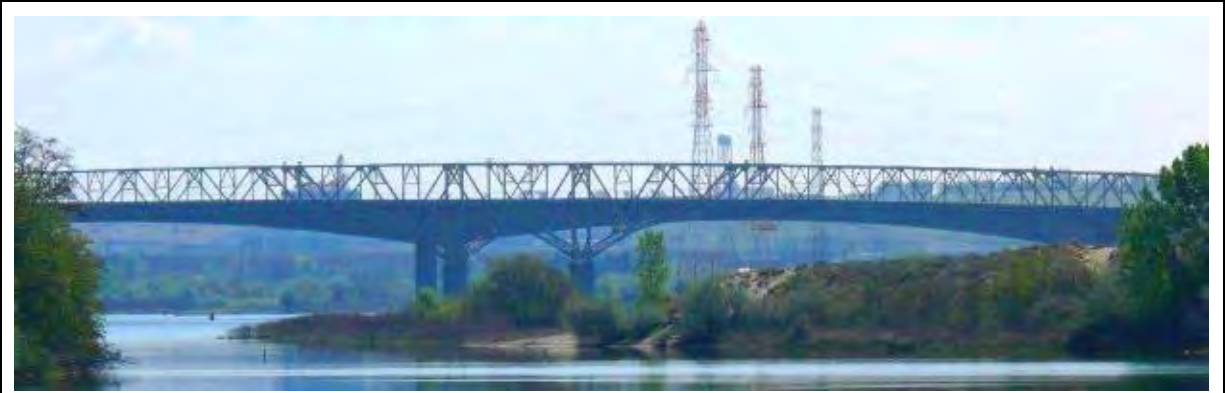
Bridge and powerlines in Benton County
