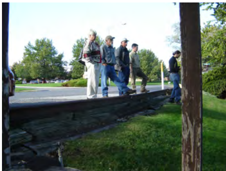
Figure 31 - The bank between the parking areas and Vista Park is hard to traverse
