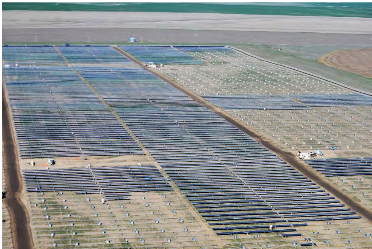
Photo 9. Construction of a USSE project in Morrow County, Oregon, March 2022. Visible infrastructure includes access roads, PV panels, posts, and associated electrical infrastructure.
