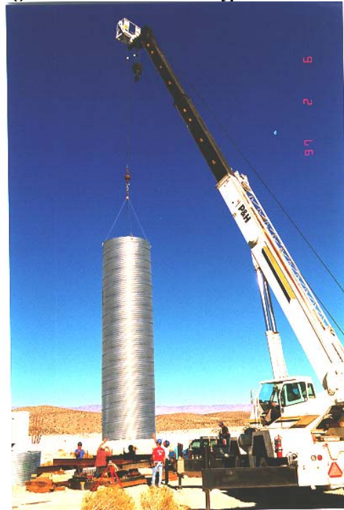
Figure 2.2.3.2-2 Mono-Pier Type Foundation
