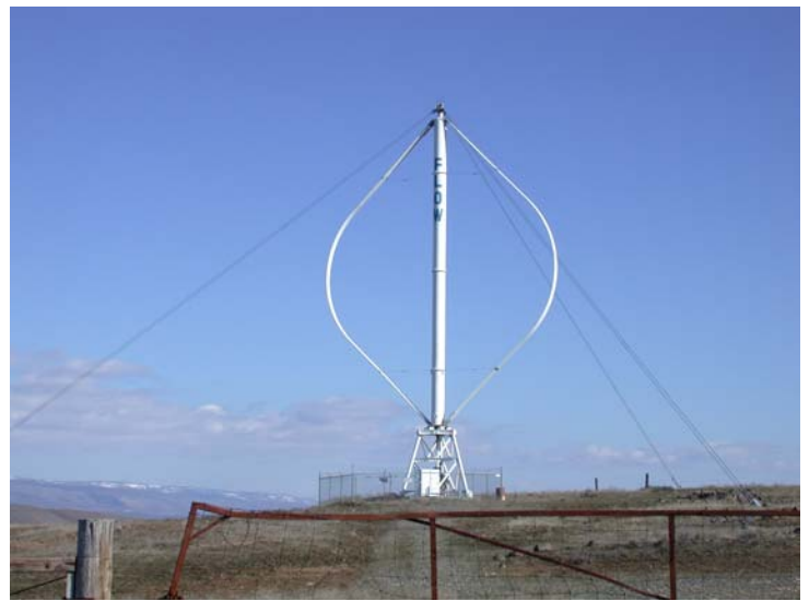
Figure 2.3.1-2 FloWind Vertical Axis (Darrieus Wind Turbine Located on Thorp Prairie, near Ellensburg WA
