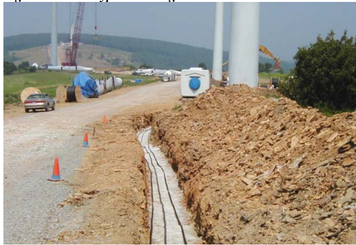
Figure 2.2.3.4-2 Typical Underground Cable Trench
