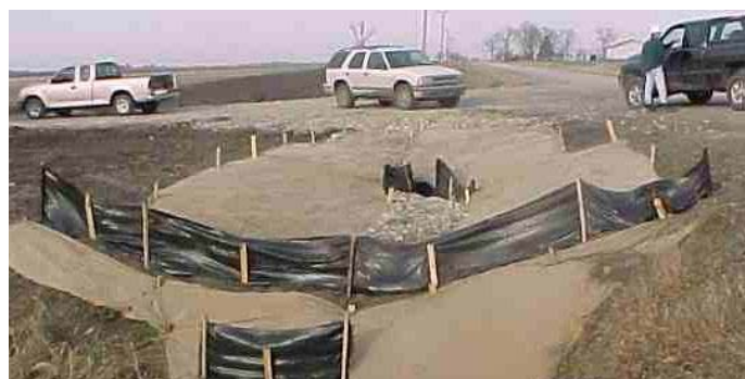
Figure 3.3.2-1 Erosion Control Blankets and Silt Fencing used for Exposed Slope Stabilization as part of a SWPPP
