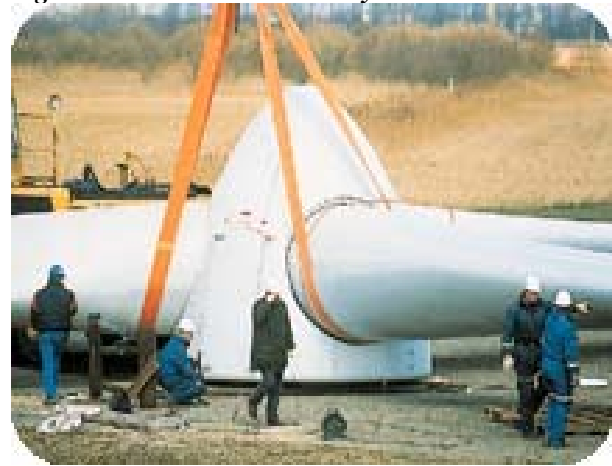
Figure 2.2.3.3-2 Rotor Assembly
