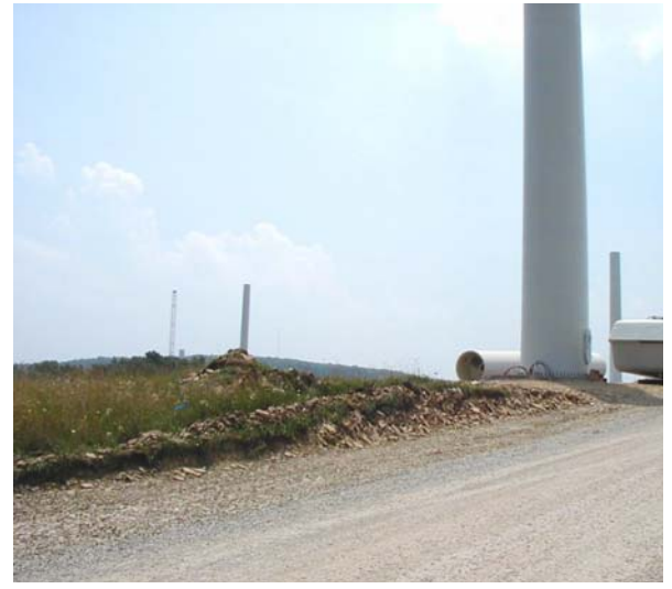
Figure 2.2.3.1-1 Typical Wind Power Project Gravel Road
