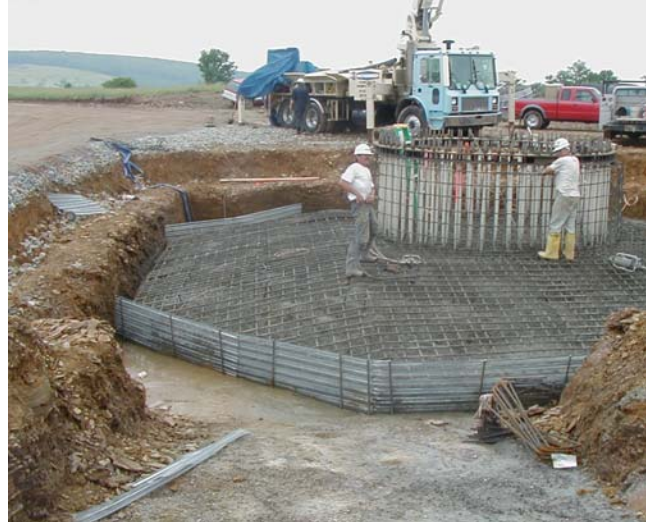
Figure 2.2.3.2-1 Spread Footing Type Foundation
