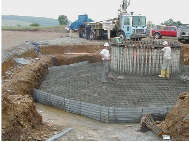
Figure 2.3.3-1 Spread Footing Type Foundation
