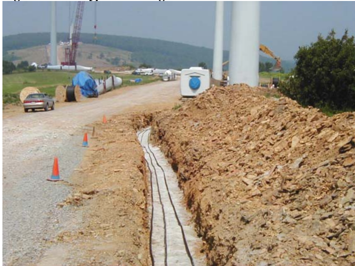
Figure 2.3.4-1 Typical Underground Cable Trench
