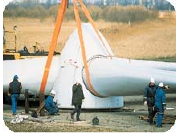
Figure 2.3.6-4 Rotor Assembly
