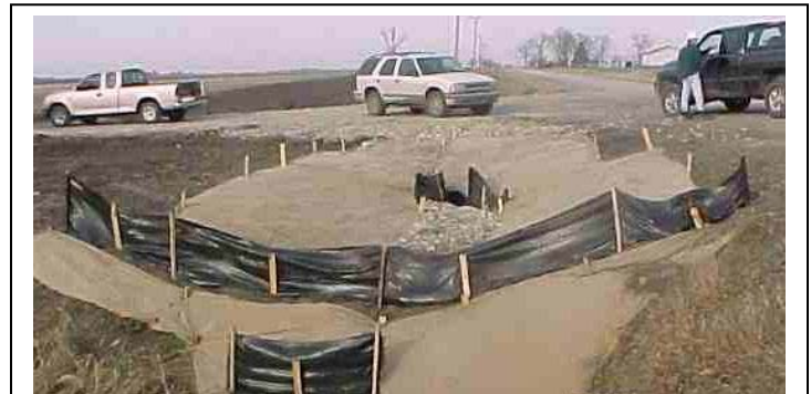
Figure 2.10.2-1 Erosion Control Blankets and Silt Fencing used for Exposed Slope Stabilization as part of a SWPPP
