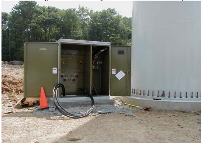
Figure 2.3.4-2 Typical Pad Mount Transformer (shown during construction before terminations landed)
