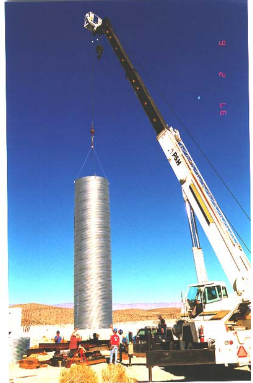
Figure 2.3.3-2 Mono-Pier Type Foundation
