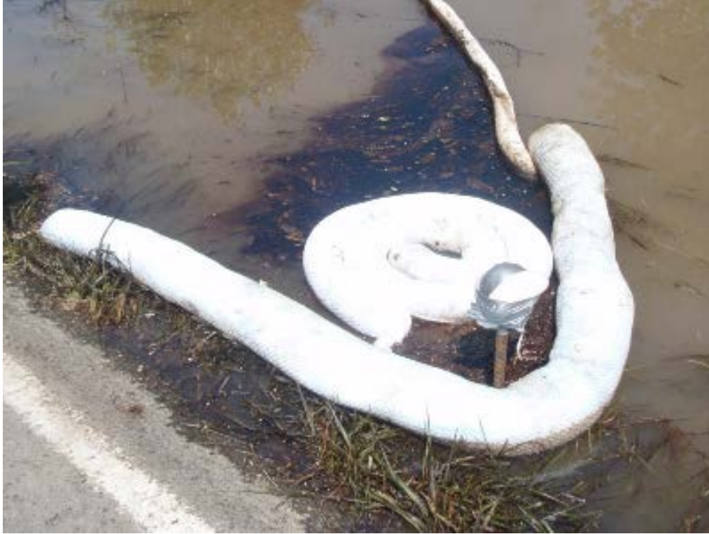
Figure 4-8. Sorbent Applied to Absorb Oil Source EPA 2015d
