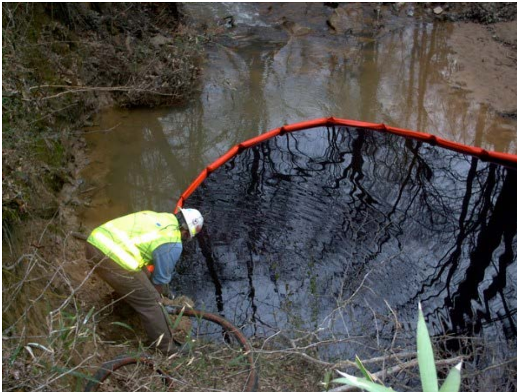
Figure 4-9. Booming and Vacuuming Oil Source EPA 2015d
